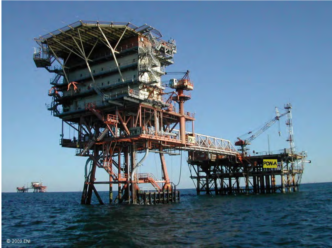
Figure 3-8 Platform “Porto Corsini MWA”, one of the platforms to be dismissed. Source: ENI
